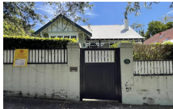
Figure 5.30 View of 119 Holt Avenue from the street, looking north.
