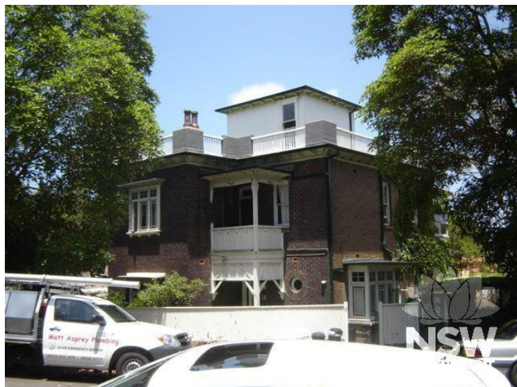
Figure 6.12 15–17 Bertha Road, Cremorne 'House'. (Source: NSW State Heritage Inventory)
