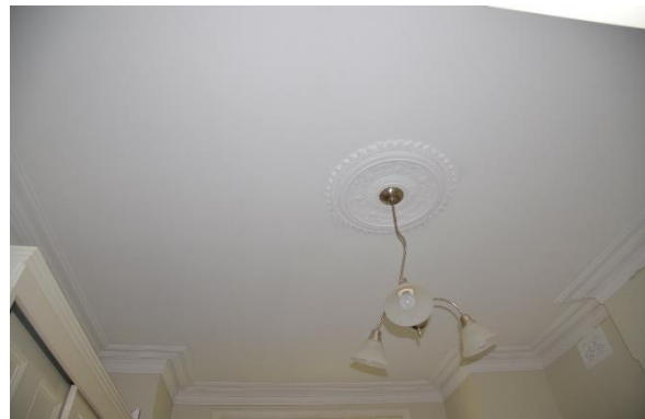
Figure 5.22 View of the plaster cornices and ceiling rose to the front bedroom.
