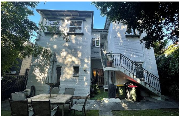
Figure 5.46 View of the rear elevation, facing south-west.
