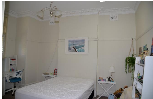
Figure 5.20 View of the front bedroom with the original fireplace sealed.
