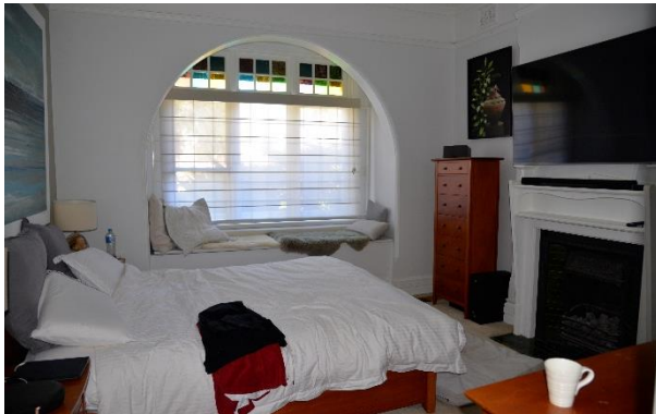
Figure 5.9 View of the original bay windows and arch with stop chamfer detailing to the front bedroom.
