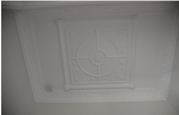
Figure 5.48 Ground floor apartment to east—original decorative plaster ceilings.
