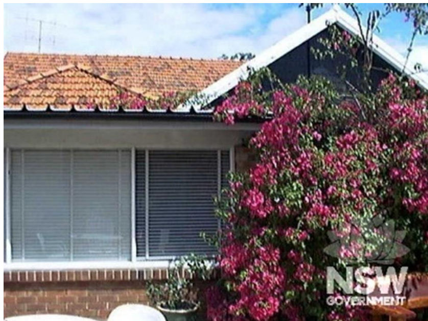
Figure 6.4 Detail of 25 Bannerman Street. (Source: NSW State Heritage Inventory)
