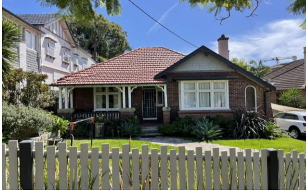
Figure 5.42 View showing the primary elevation of 123 Holt Avenue, looking north.
