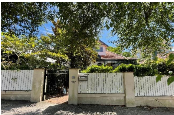
Figure 5.17 View of 117 Holt Avenue from the street, looking north.
