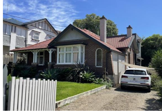
Figure 5.43 View showing the eastern elevation, roof form and temporary car shade, looking northwest.
