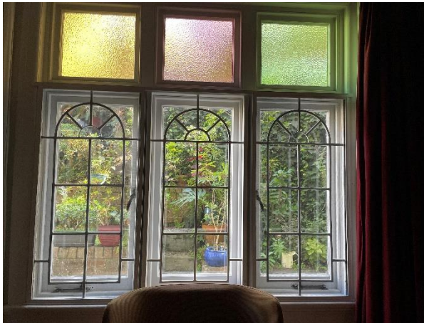
Figure 5.56 First floor apartment to west—original timber-framed casement windows with stained glass.
