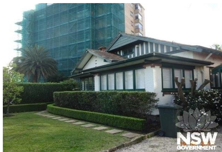
Figure 6.2 Primary façade of 24 Cranbrook Avenue. (Source: NSW State Heritage Inventory)
