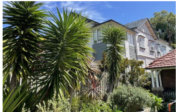
Figure 5.45 View showing a detail of the upper storey of the eastern elevation. The enclosed balcony, with timber detailing, is visible.
