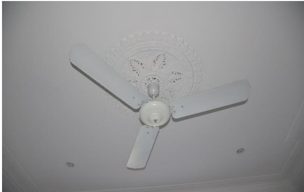
Figure 5.7 Original plaster ceiling roses to the front section of the dwelling.
