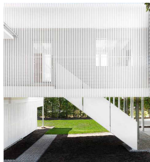
BS: PRIVACY BATTEN SCREEN (BALCONY AT THE REAR) POWDERCOATED IN COLOUR PT2
