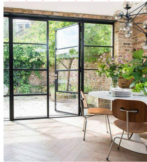
NOTE: WINDOWS AND DOORS (FACING BACKYARD) FR1: METAL FRAME DOOR AND WINDOWS FRAME COLOUR: POWDER COATED IN COLOUR PT1
