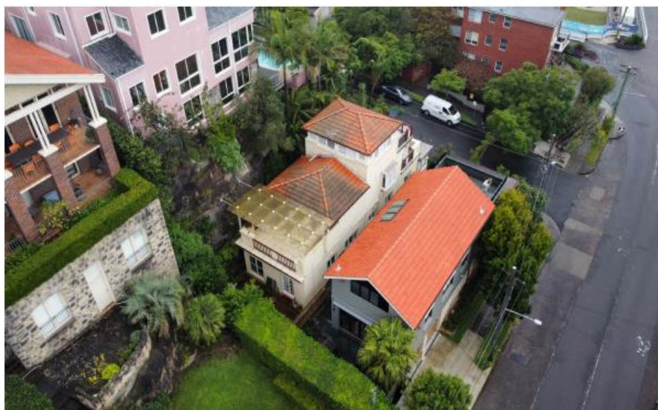
Figure 12. Aerial view of the site and adjoining buildings from the rear
