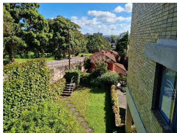
Figure 12. Existing western courtyard adjacent to Park Avenue
