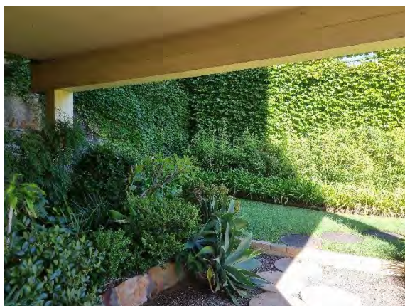
Figure 9. Existing western side undercroft and courtyard below Park Avenue
