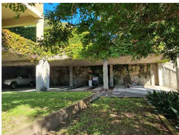
Figure 11. Existing excavated parking area
