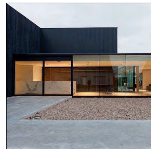
AFG ALUMINIUM FRAMED GLAZING DULUX DURATEC ETERNITY CHARCOAL PEARL SATIN OR SIMILAR
