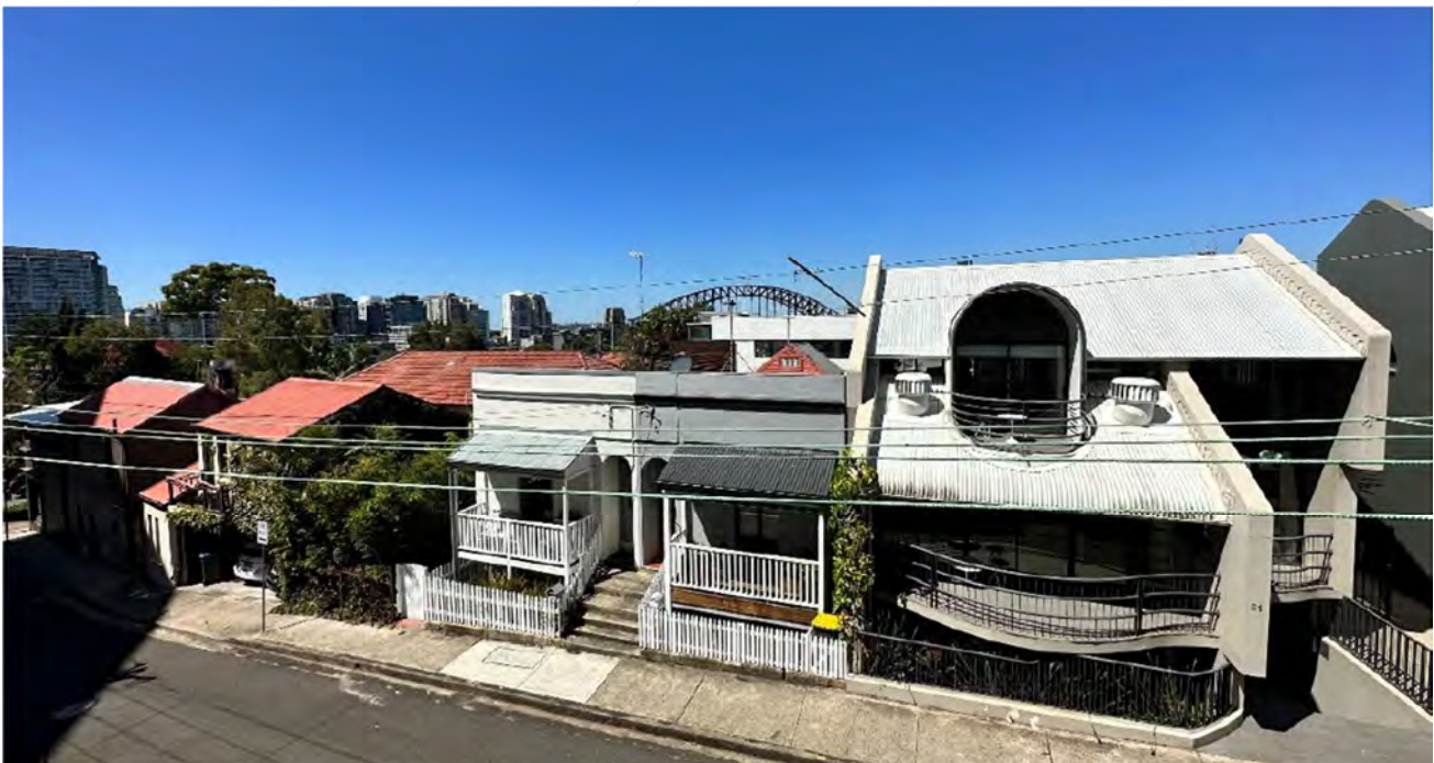
Figure 5 Existing View Corridor from First Floor Level (Standing) – 62 Victoria St. Source: North Sydney Council
