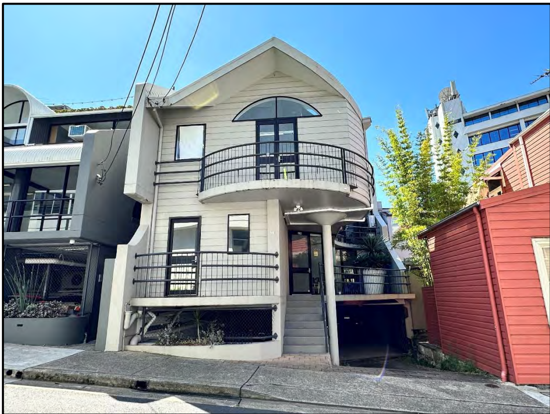
Figure 28: Rear of commercial building at No. 61 Victoria Street (view from Mitchell Street)
