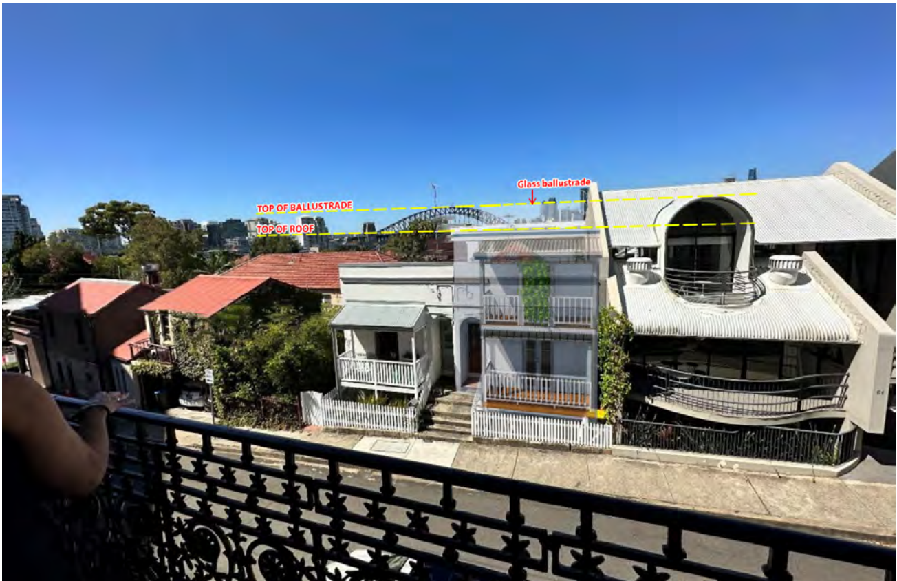
Figure 12 Proposed View Corridor from First Floor Level (Standing) – 64 Victoria St. Source: Photomontage Markey Group 2023
