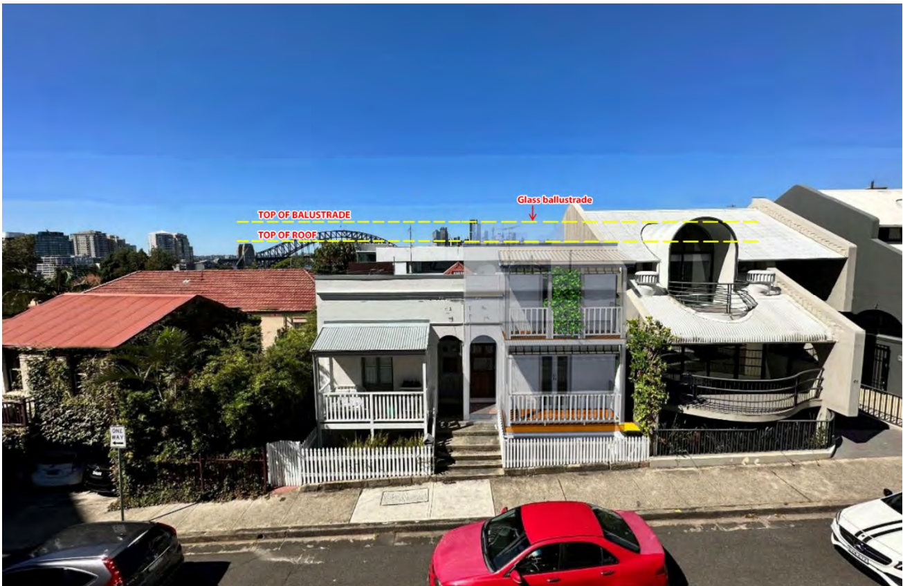
Figure 13 Proposed View Corridor from First Floor Level (Standing) – 66 Victoria St. Source: Photomontage Markey Group 2023
