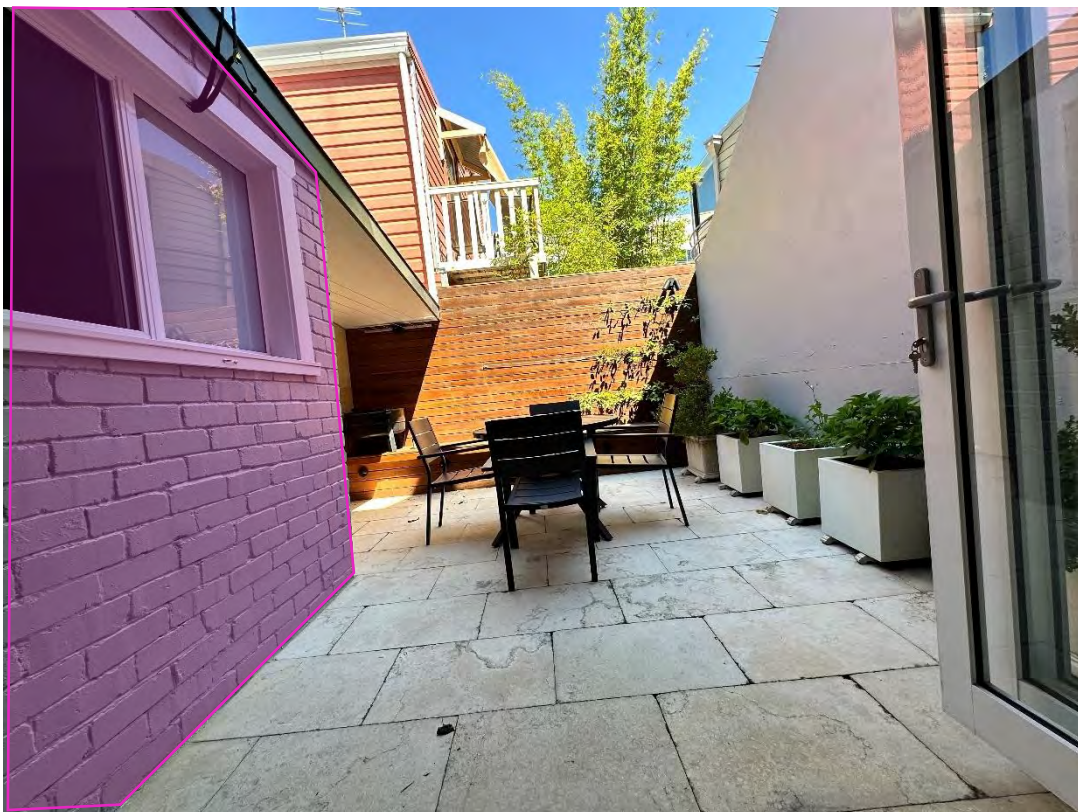
Figure 21: Open rear courtyard area with roofed clothes drying area and lower ground floor bathroom (shaded in pink)
