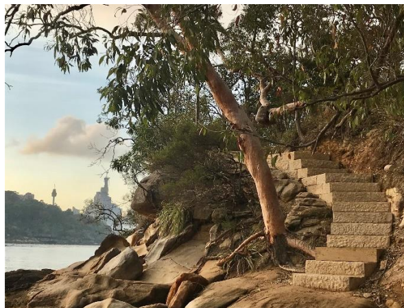
New sandstone stairs to the foreshore
