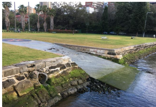
Milson Park boat ramp is now longer, wider and the slope is less steep
