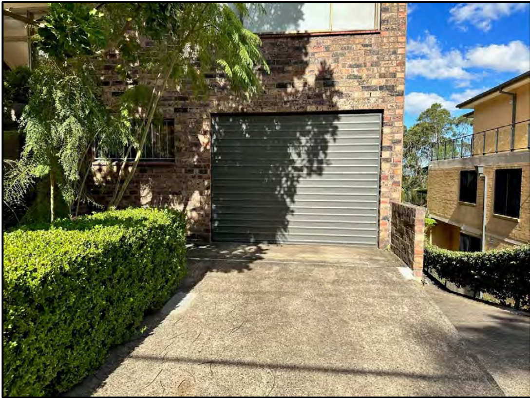
Figure 12: Front of garage of Unit 6 – to be converted into a multi-media room
