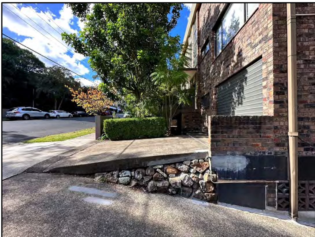
Figure 11: Existing driveway to access garage of Unit 6
