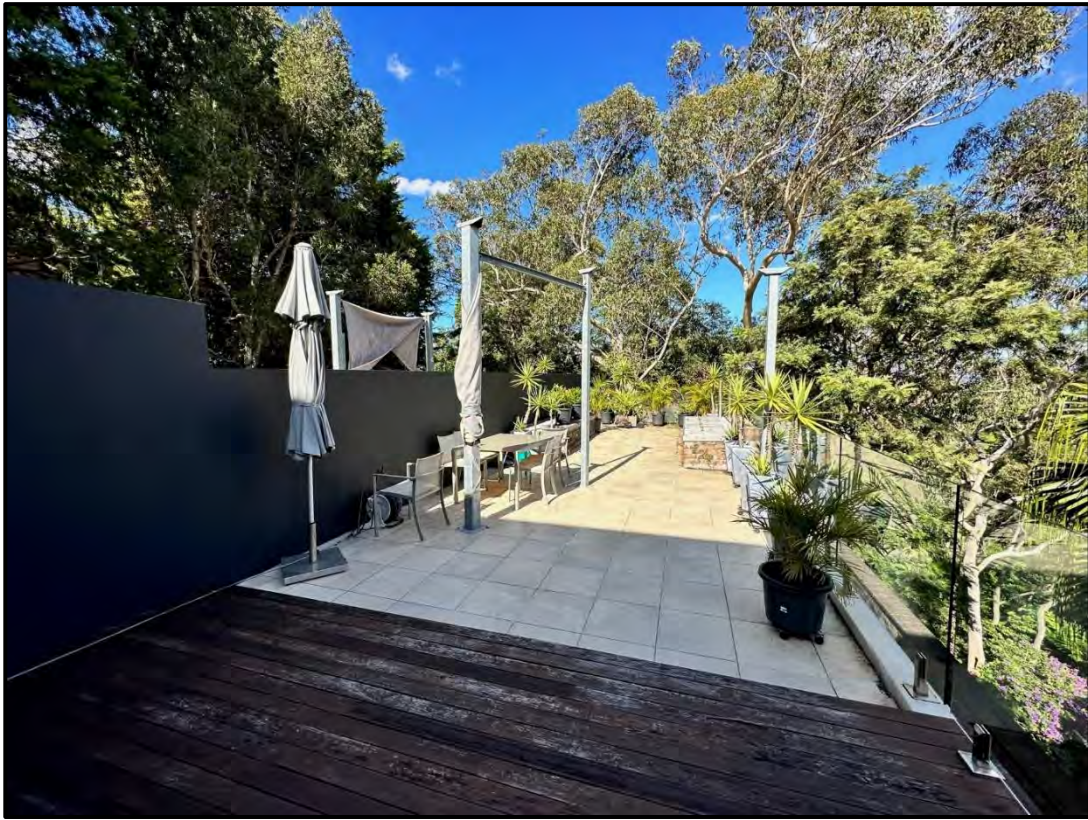
Figure 16: Existing roof terrace with timber deck (currently unroofed) – view to the south
