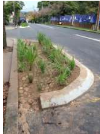
Rain gardens – Union Street, McMahons Point
