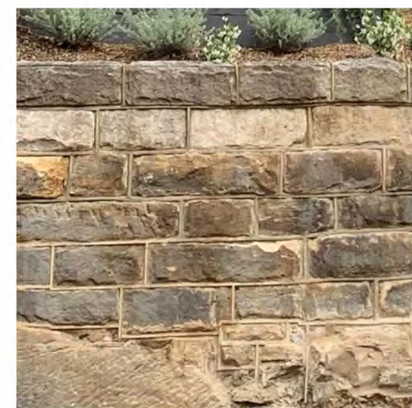
ST SANDSTONE CLADDING (REUSED EXISTING)
