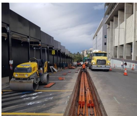
Typical electrical trenching
