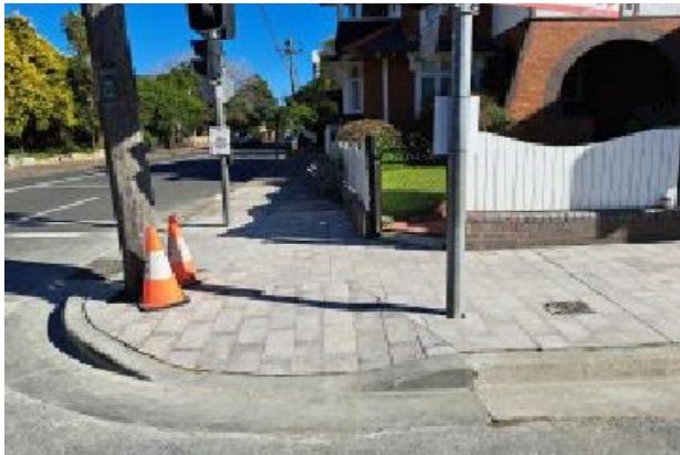
Streetscape upgrade corner Wycombe Rd and Yeo St outside no. 144
