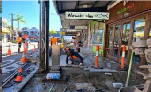
Streetscape upgrade outside 161 Wycombe Road looking north.
