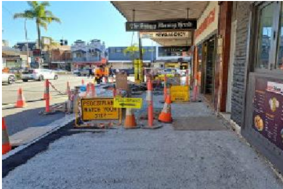
Streetscape upgrade near corner Wycombe Rd and Military Rd looking north
