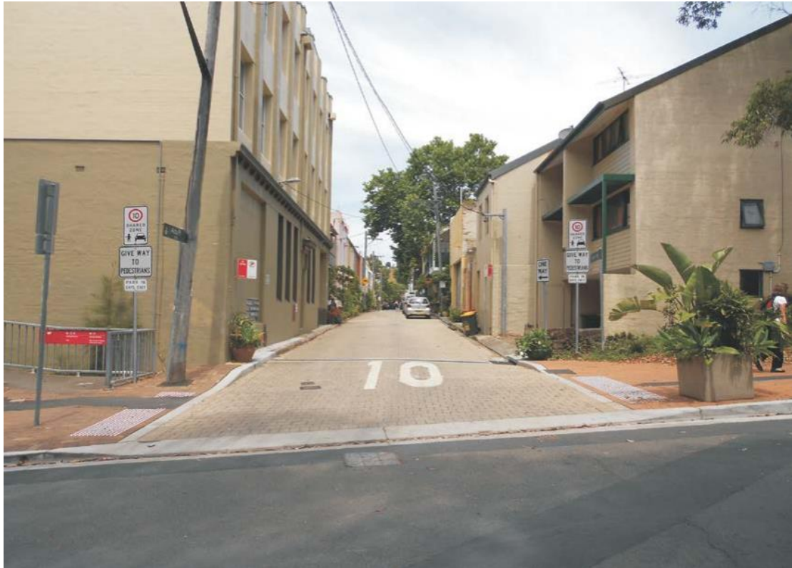
Figure 6. Typical layout of a Category 1 Shared Zone with retaining kerb and gutter as shown in RMS Technical Direction TTD 2016/001.
