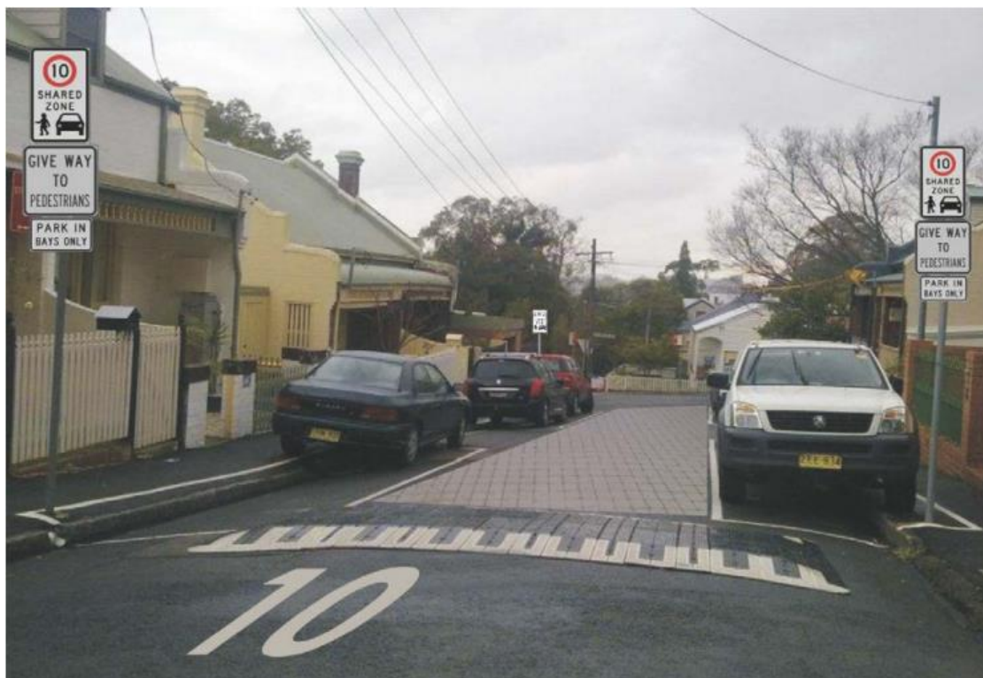
Figure 7. Typical layout of a Category 2 Shared Zone with footpath parking and traffic calming devices as shown in RMS Technical Direction TTD 2016/001.
