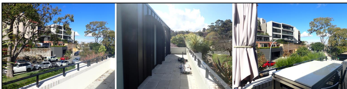
Figures 18, 19 & 20 – Photos from various points of the Unit 602 balconies subject to the proposed awning
