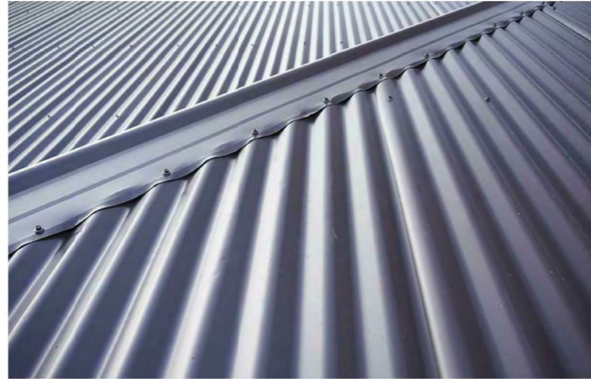
MR METAL ROOFING (AND ASSOCIATED FLASHING, GUTTERS AND DOWN PIPES)
