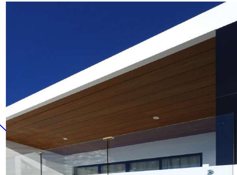
Timber soffit, white render and glass balustrade to balconies
