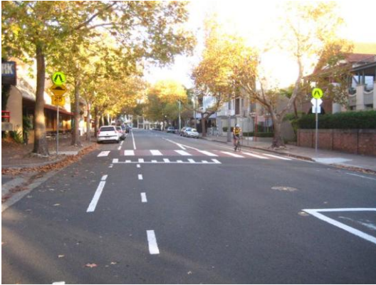
Figure D6: Ridge Street (looking west)
