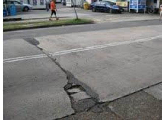
Figure D9: Spofforth Street near Brierley Street (looking west)
