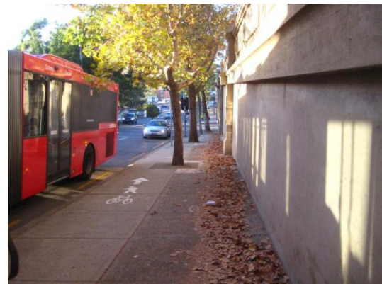
Figure D13: Pacific Highway Shared Path (looking south)
