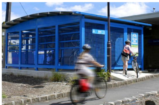
Figure 6.14: East Malvern Railway Station, Victoria
