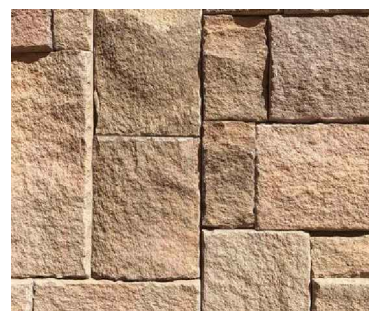
ST SANDSTONE CLADDING
