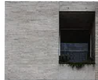
BR1 STANDARD 76MM BRICK IN STACK BOND, GHOST GREY, FLUSH JOINTS
