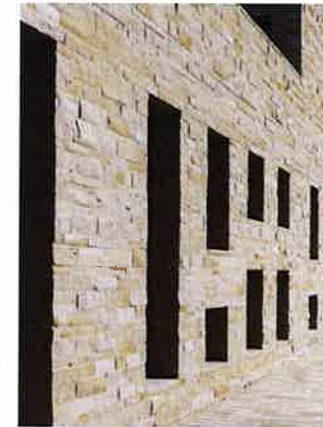
S11 STONE BLOCKS, DRY PRESS JOINTS
