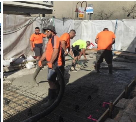
Drainage pipe installation at Bligh Street Main concrete slab poured
