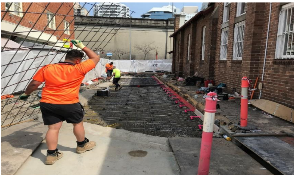
Main concrete slab and drainage in progress
