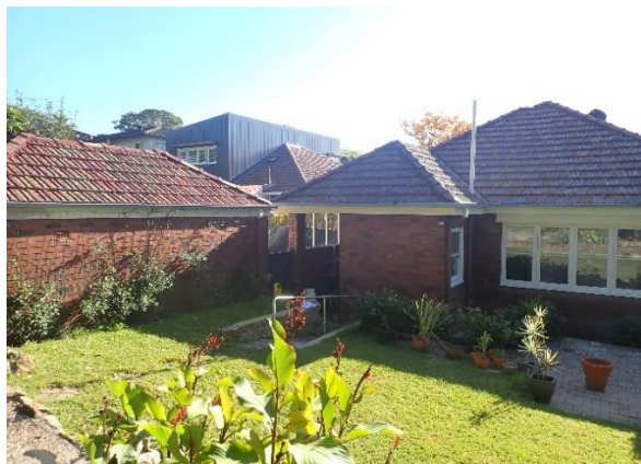
Figure 35 – Photo of the adjoining property No. 5 Ryries Parade
