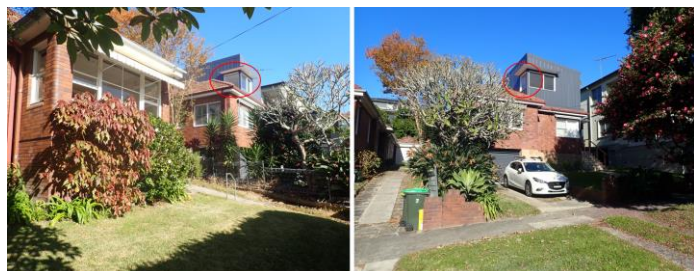
Figures 36 & 37 – Photos of the corner north facing window on the first floor (circled in red) of the adjoining property No. 5 Ryries Parade
