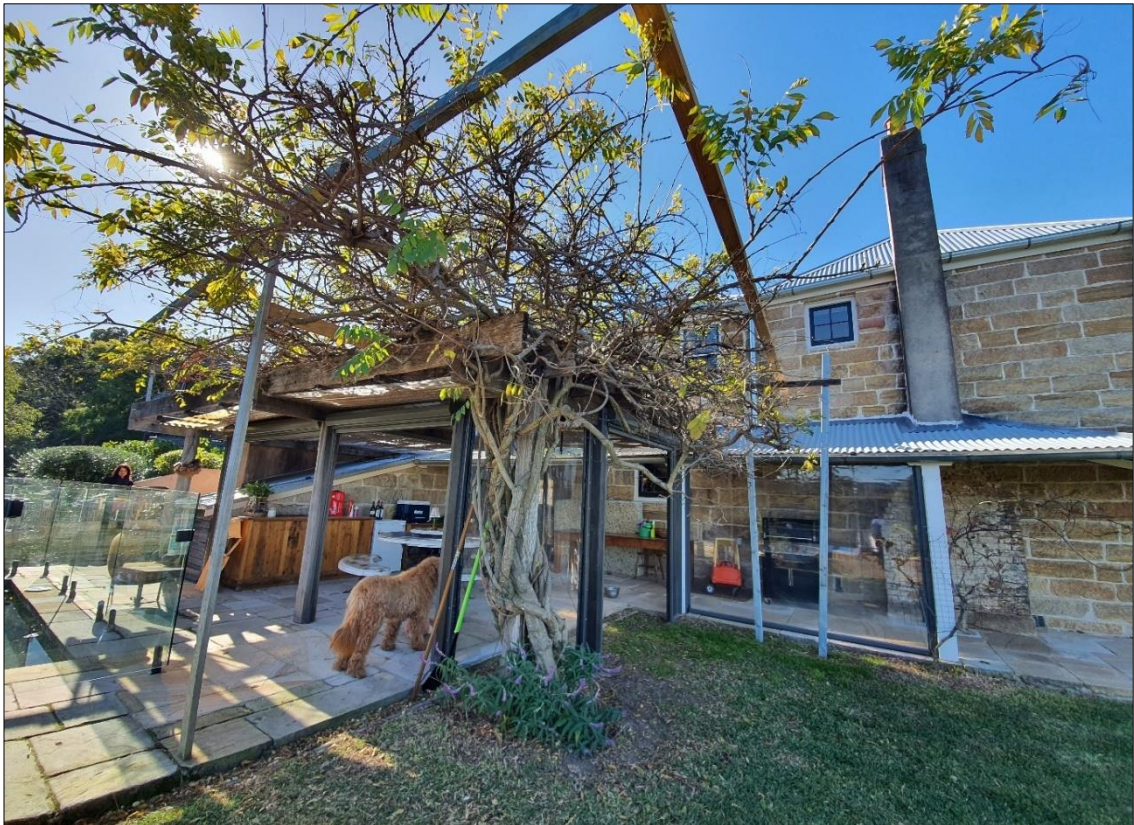
Figure 9e: View towards the rear elevation of the existing dwelling from the backyard
