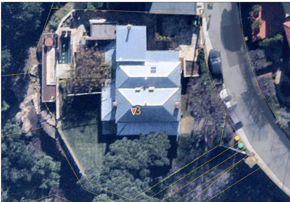
Figure 9y: Unauthorized skylight installation sometime between 21/11/2022 – 9/1/2023 (NearMaps accessed on 7 September 2023)
