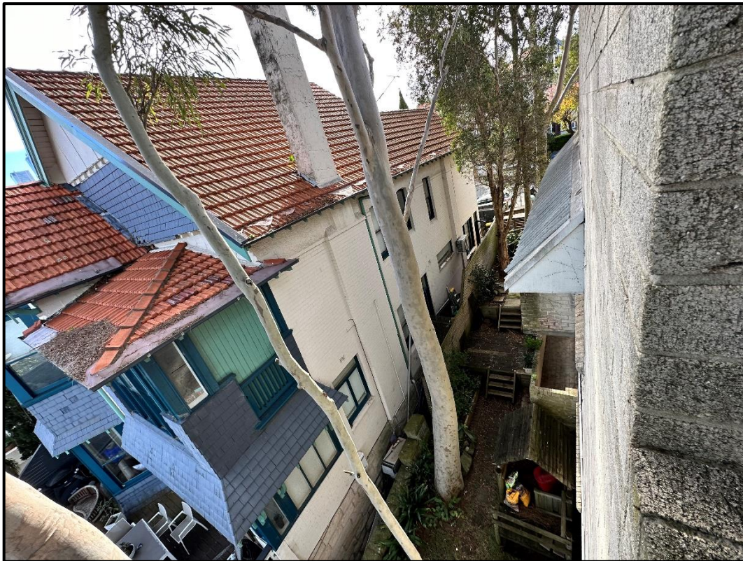
Figure 16: View of western side setback from rear of Unit 5 (penthouse apartment)
