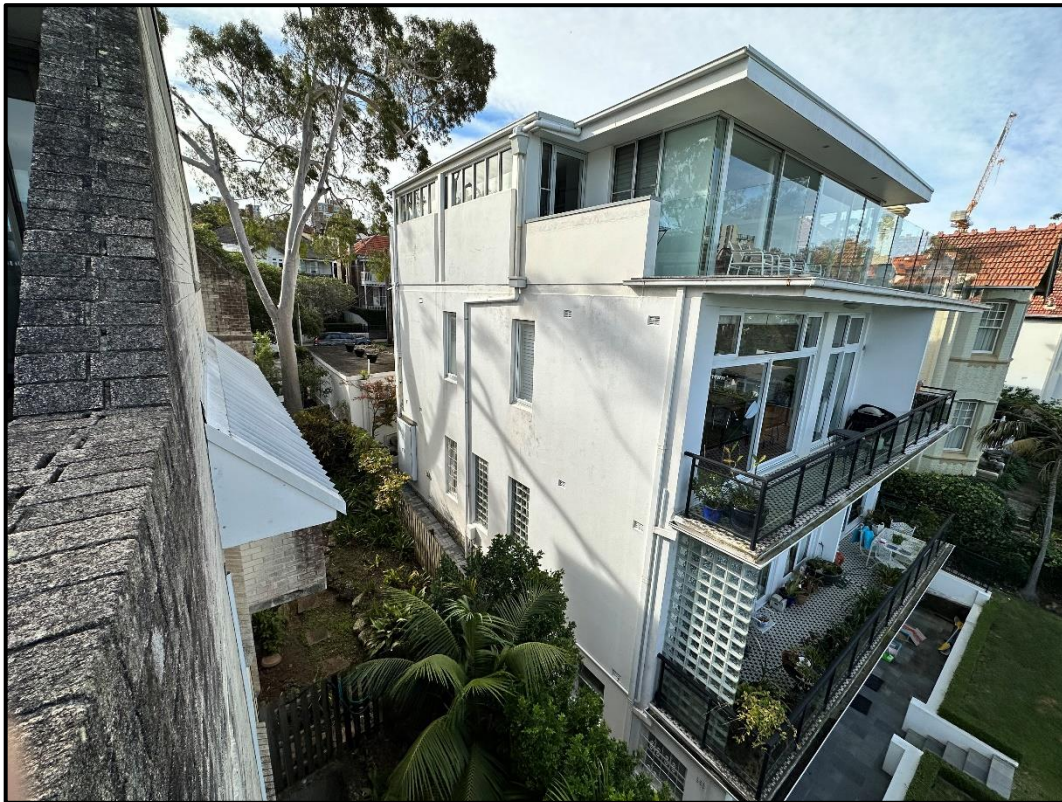
Figure 14: View of eastern side setback from rear of Unit 5 (penthouse apartment)
