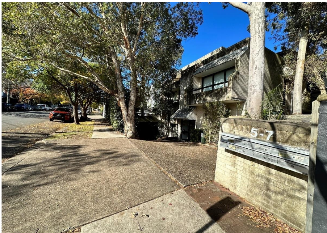
Figure 9: Front of existing building – showing mail boxes and driveway leading to basement
