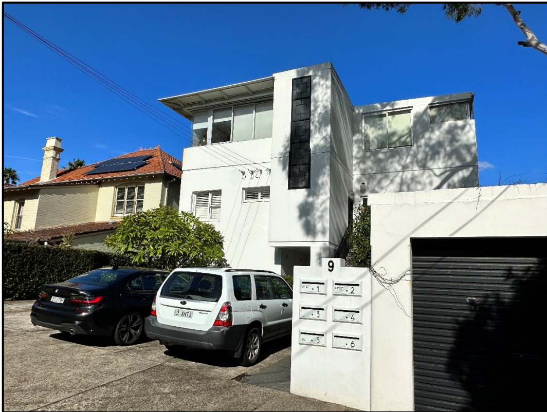
Figure 25: Residential flat building at No. 9 Lower Wycombe Road
