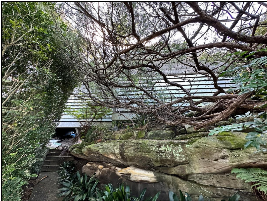
Figure 18: View of southern elevation of existing building
