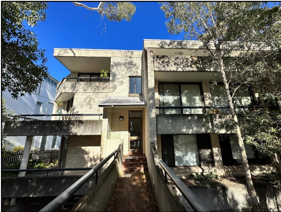
Figure 10: Front of existing building – showing pedestrian bridge and entry lobby for Units 1-5
