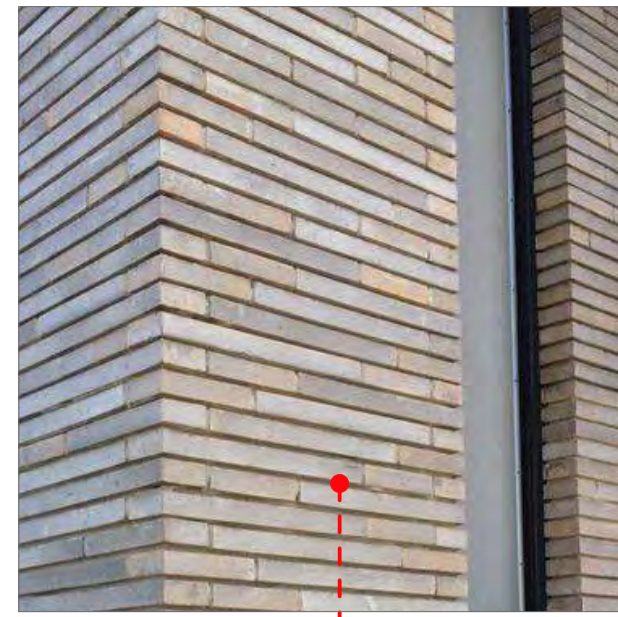
ST1 TILED FINISH 01 AUSTRAL BRICKS - PALE GREY - SAN SELMO LIVENZA RAW OR SIM.
