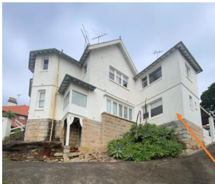
Rear later addition
