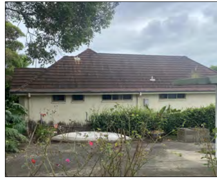
Image of 3 Shellcove Rd overlooking site
