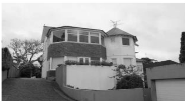
The primary façade showing southern faceted bay addition c 1930s. Image: John OultramHeritage Impact Statement August 2023
