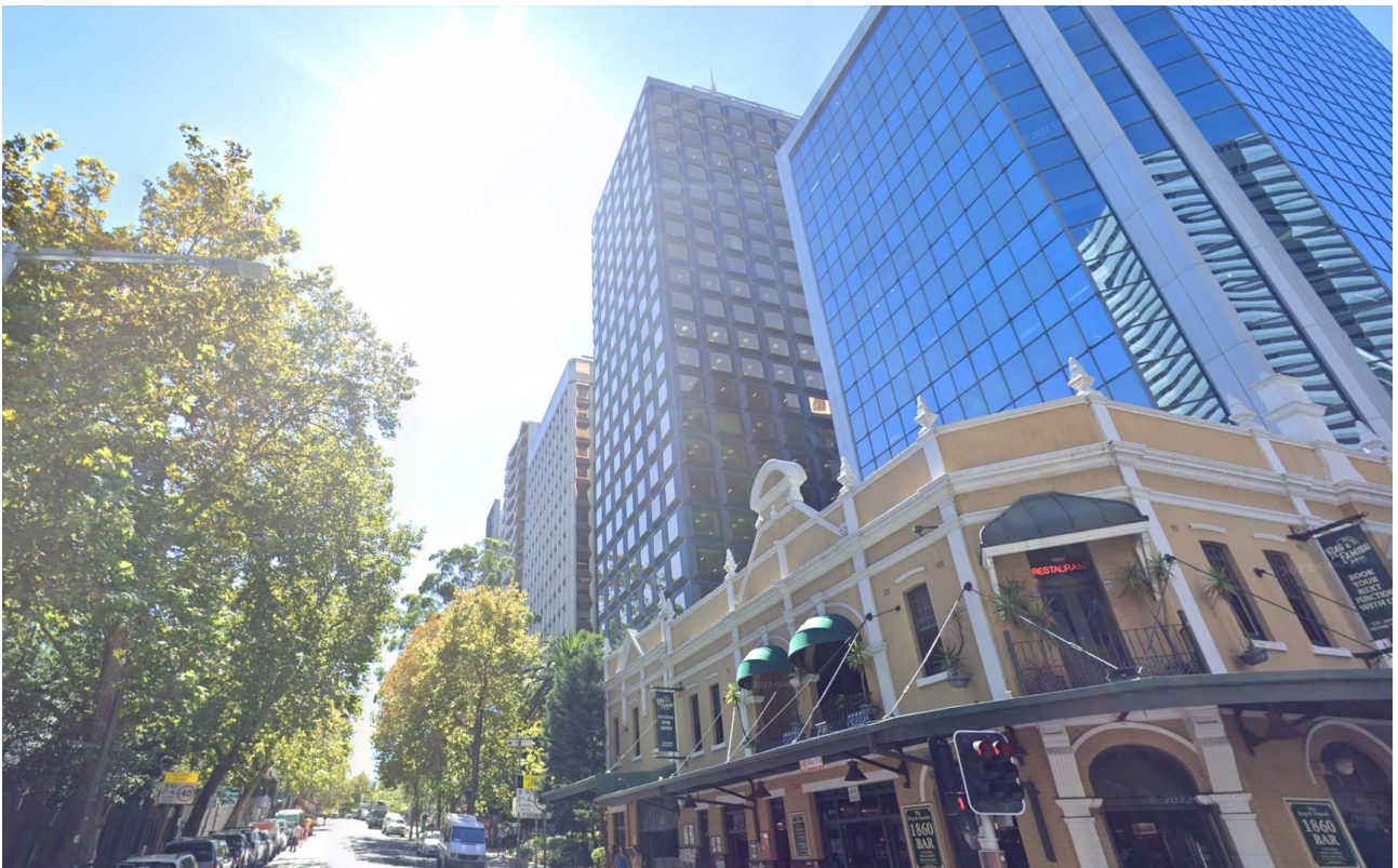
Figure 6 – View north along Miller Street showing the subject site within its context.
