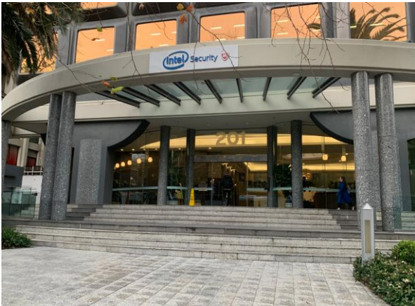
Figure 4 – View to the existing primary entry from Miller Street.
