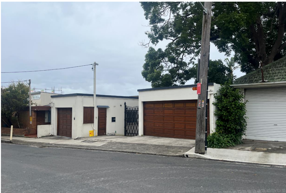
Figure 8: No. 186 Kurraba Road as viewed from public domain in an easterly direction
