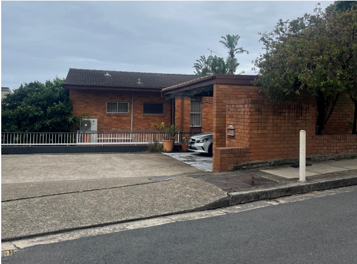
Figure 7: Nos. 184B Kurraba Road as viewed from public domain in an easterly direction
