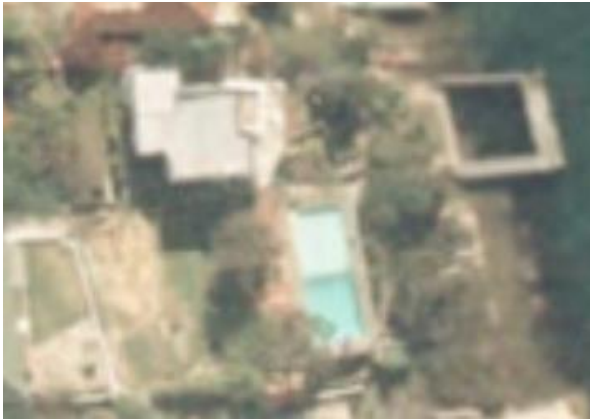
Figure 5 – Aerial imagery of 186 and 188, 1986. Note first floor extension.
