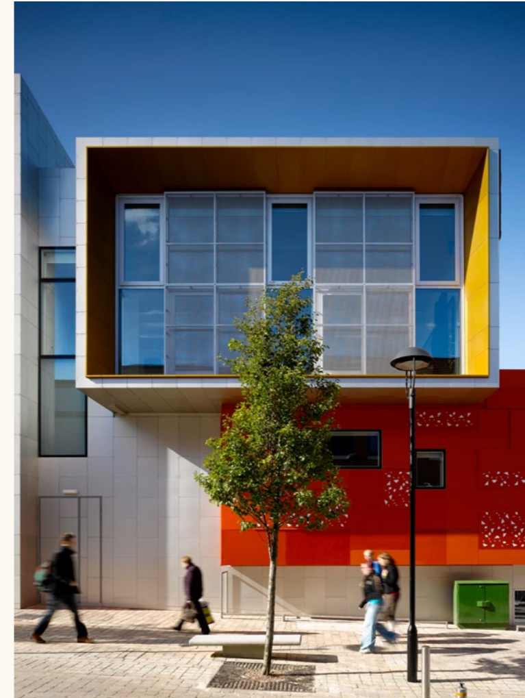
Jacqueline Poncelet and Richard Layzell with Ellis Williams Architects, Cornerstone Arts Centre, Didcot, UK (image - Ellis Williams Architects)
