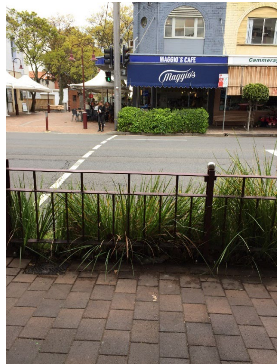
Figure 20 Protection barriers The design of protection barriers for pedestrians on busy Miller Street, Cammeray successfully integrates high quality design and safety.
