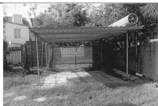
View of carport towards Wellington Lane
