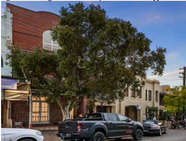
Figure 9: View of the front elevation. From Blues Point Road.
