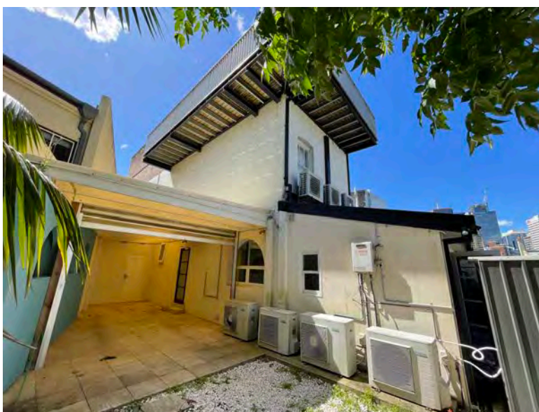
Figure 6: Looking towards the garage along the Southern elevation of the subject site.
