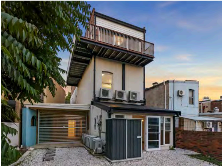
Figure 11: Looking towards the southern and eastern elevations of the rear wing.
