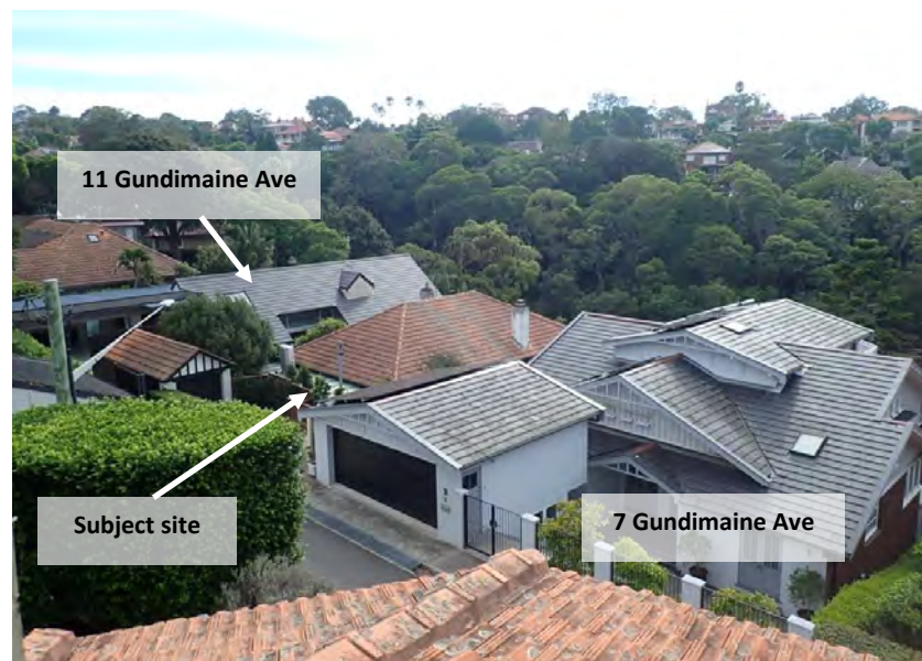
Figure 15: The subject site and adjoining properties as seen from an adjoining property to the south-west
