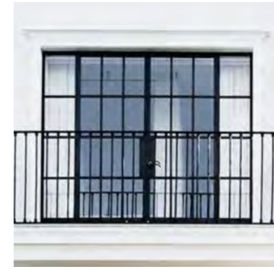
4 - ALL EXISTING AND NEW WINDOWS TO HAVE BLACK PAINTED TIMBER FRAMES. BLACK STEEL BALUSTRADES
