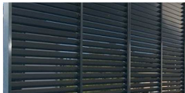
POWDERCOATED ALUMINIUM WINDOW FRAMES AND EXTERNAL LOUVRE SCREENS: DULUX COLORBOND MONUMENT - TO MATCH EXISTING WINDOWS
