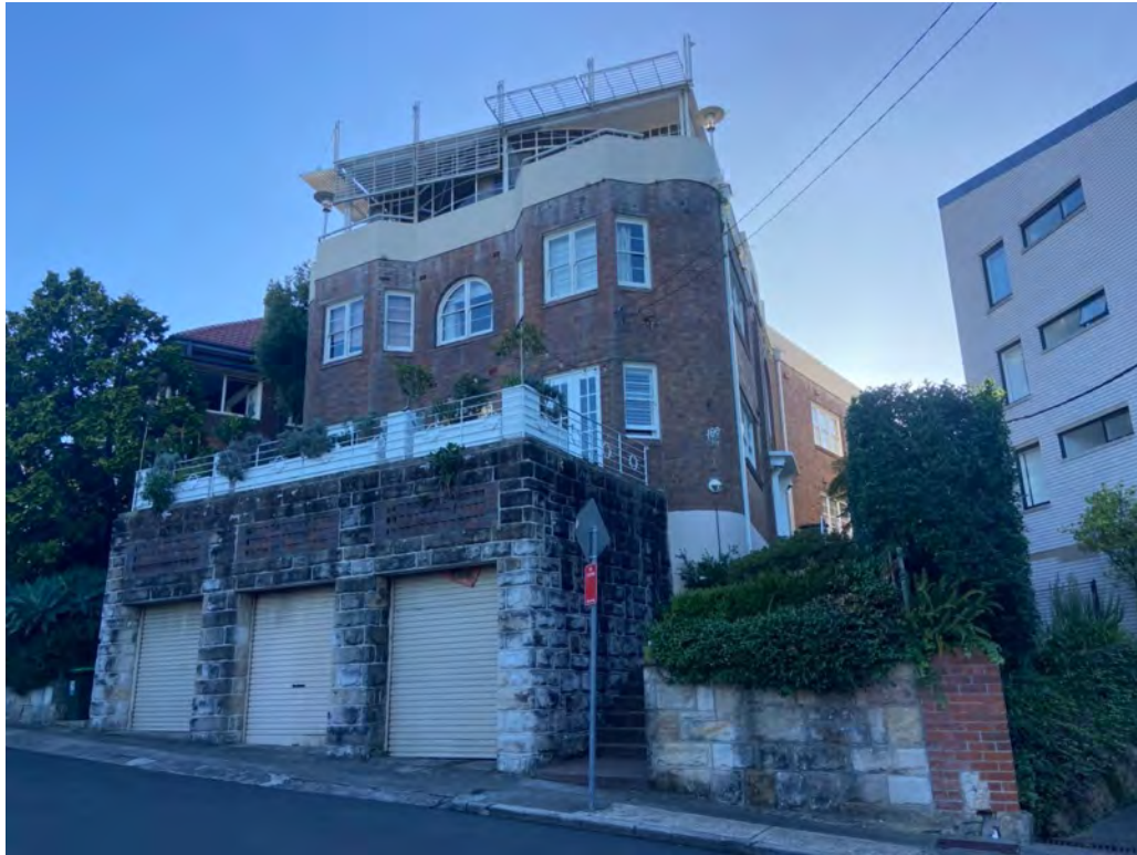
Figure 18: The view from directly outside of the site.
