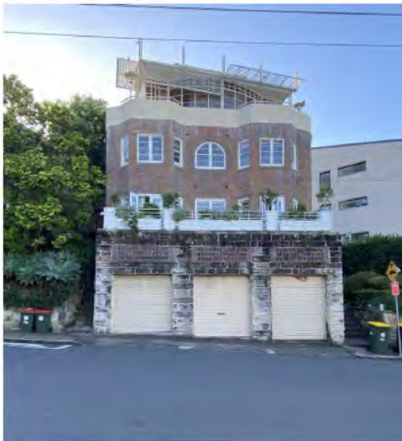
Picture 8 Existing Street View
