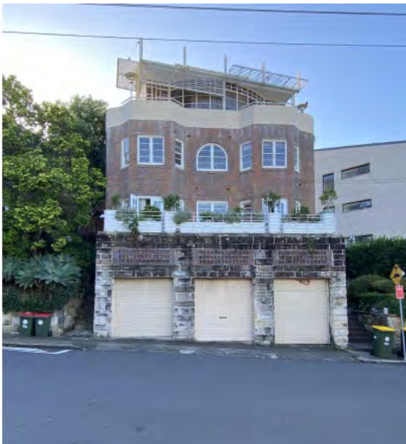
Picture 12 Existing Street View
