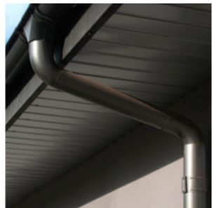
3 Half round metal gutter & downpipes
