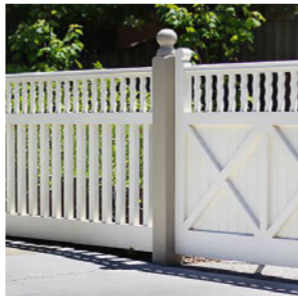
5 Painted Timber Gate & Fence
