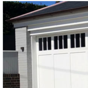
7 Painted Timber Garage Doors
