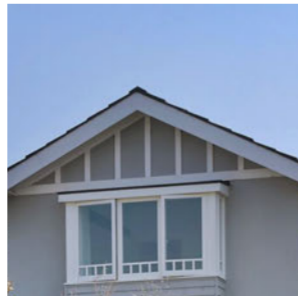
4 Timber federation battens
