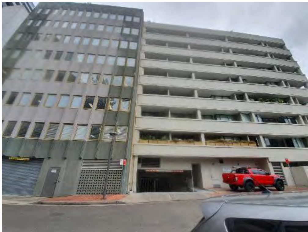
Figure 12: View from subject site (rear) to the neighbouring buildings south
