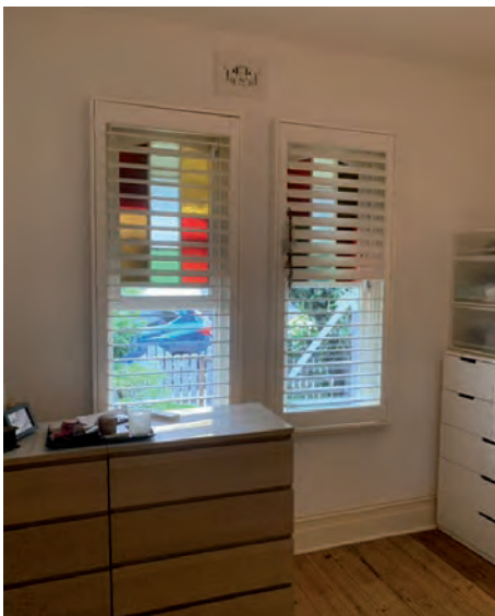
Figure 3.9 view from within bedroom looking towards oak Street through the intact timber double hung window.
