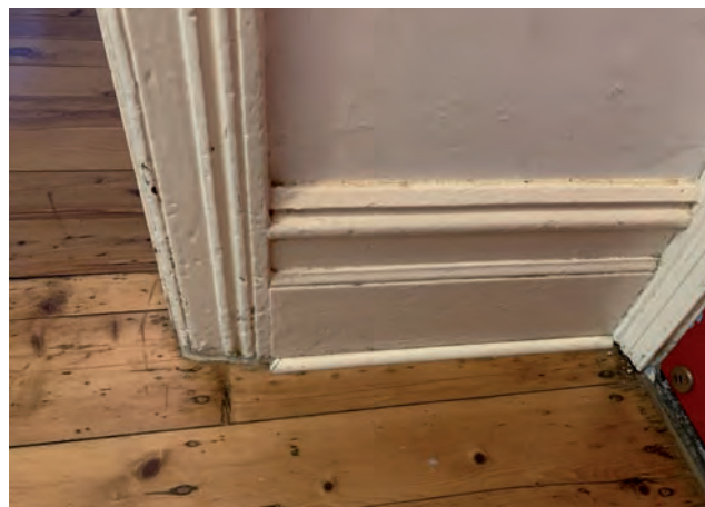
Figure 3.5 Original floorboards, skirting and architraves survive. Source: Studio Aalma
