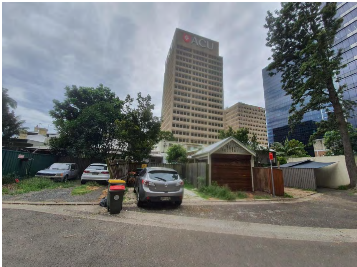
Above: Laneway elevation showing bin storage area behind car on the left of the yellow sign on timber fence
