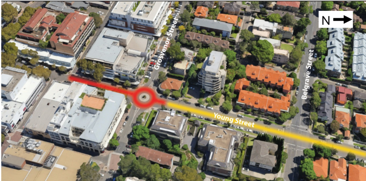
Image 1. The project site (red section) is the final link of the Young Street Extensions (yellow line)
