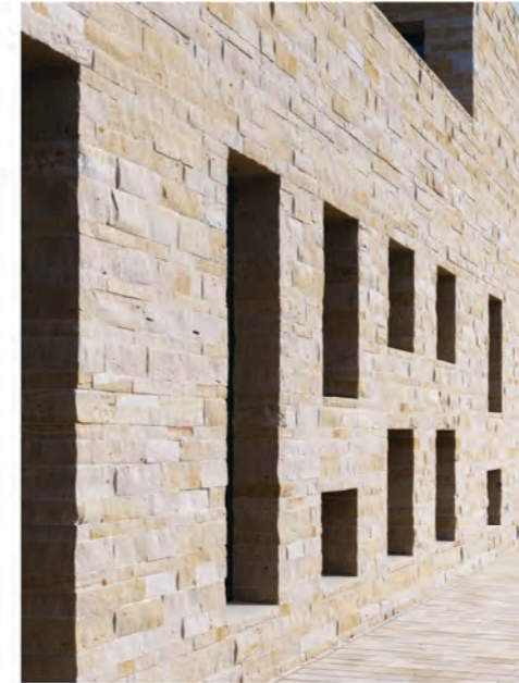
ST1 STONE BLOCKS, DRY PRESS JOINTS
