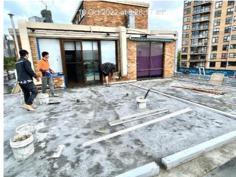
EPOXY APPLIED TO SUNROOM AND TERRACE AREAS, SCREED AND FALL WAS CREATED (10 OCT 2022)
