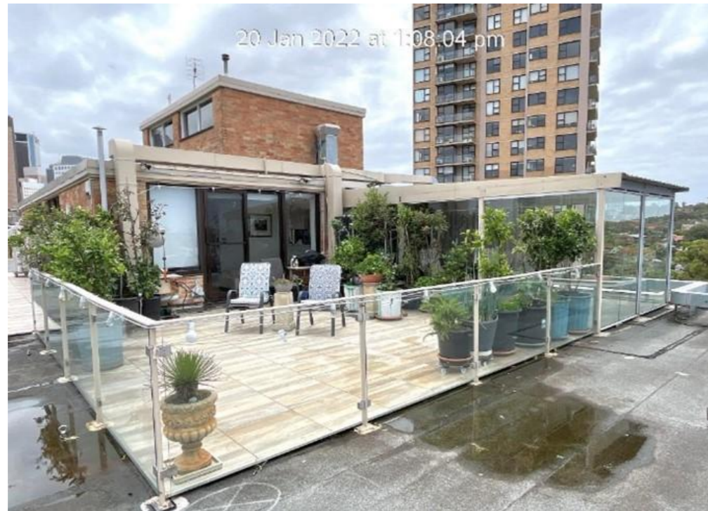
BEFORE STRATA WATERPROOFING - SOUTH EAST VIEW - EXISTING TERRACE/ DECK (20 JAN 2022)
