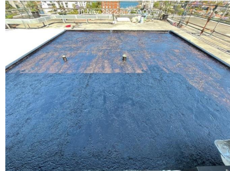
BITUMEN APPLICATION ON THE SUNROOM AND TERRACE (10 NOV 2022)
