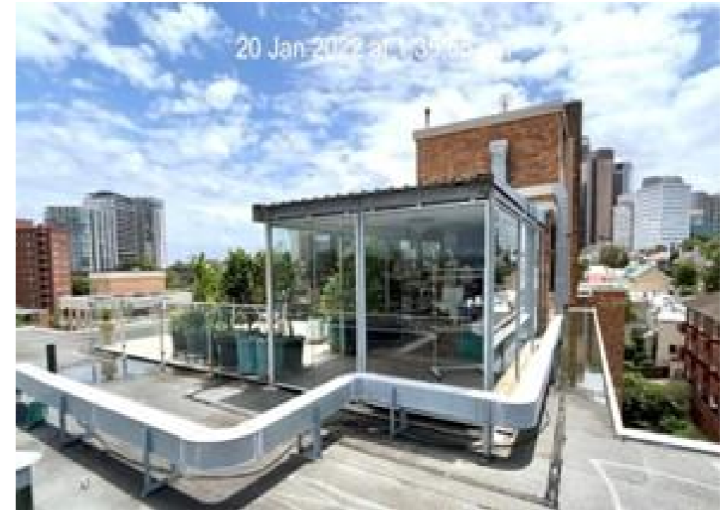
BEFORE STRATA WATERPROOFING - NORTH EAST VIEW - EXISTING SUNROOM (20 JAN 2022)
