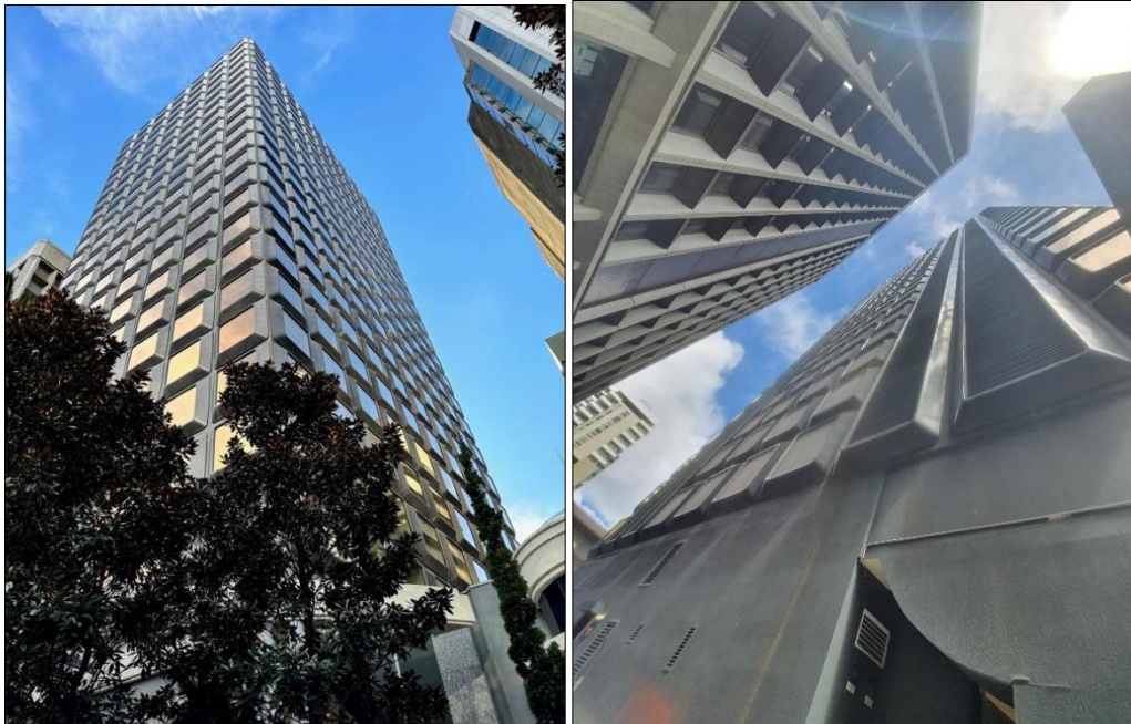
Figure 7c (left): SW view of existing building; Figure 7d (right): Northern elevation of building with 4 columns of existing vertical louvers
