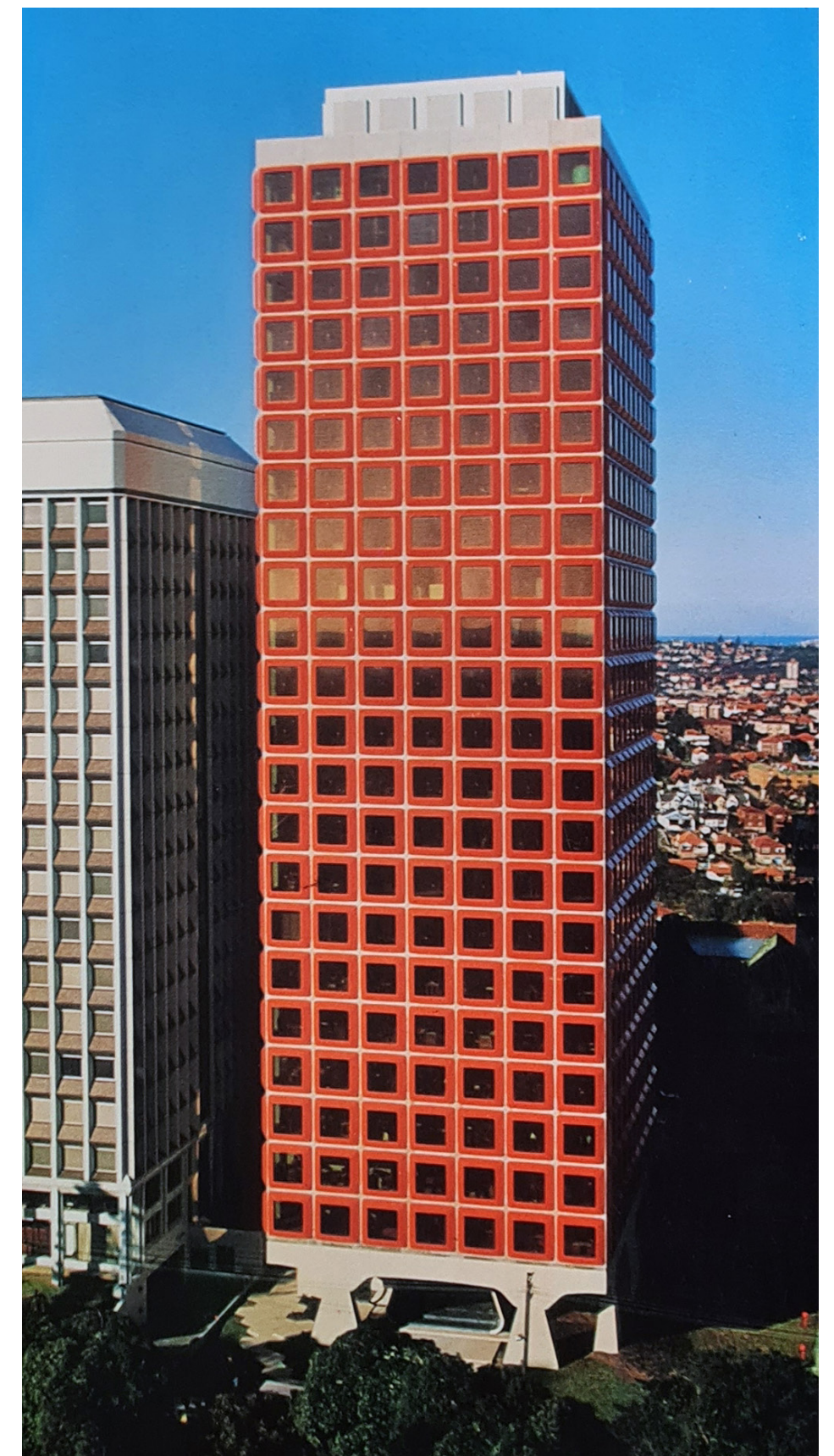
Original Building - Orange Shrouds + Bronze Glass - Miller Street
