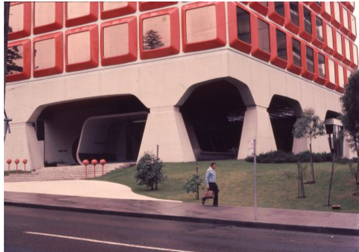
Original Building - Entry and Lobby Columns
