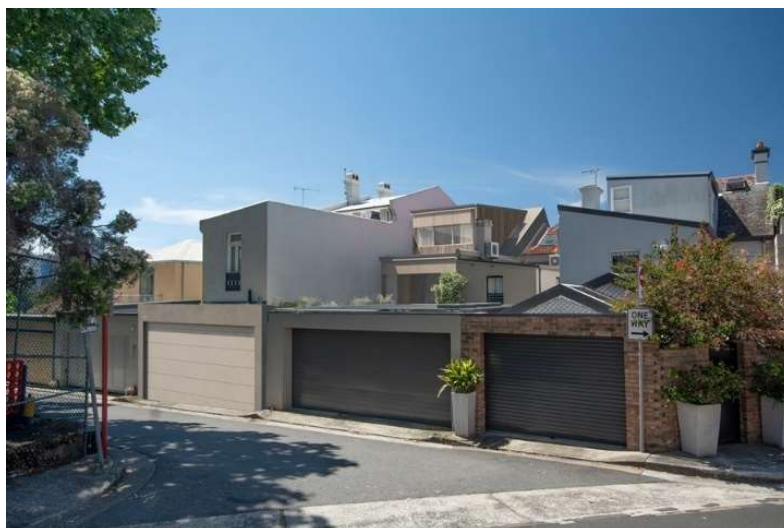
Figure 5 – Render of the altered terrace and its compatibility with its adjacent context as viewed from Crescent Place
