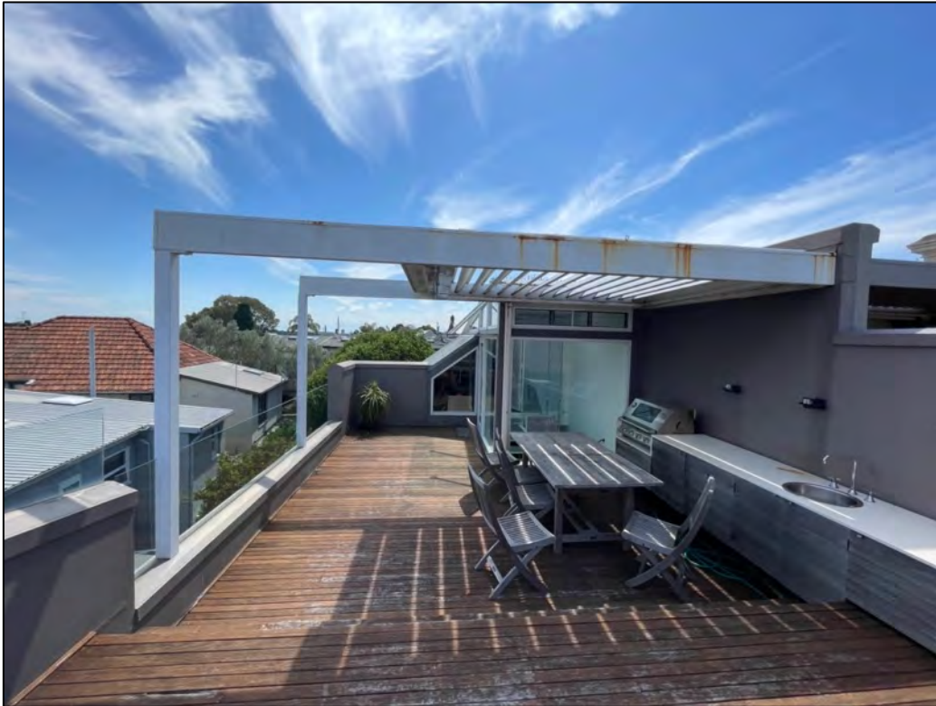
Figure 6: Rooftop area of No. 2 Waiwera Street, facing west.
