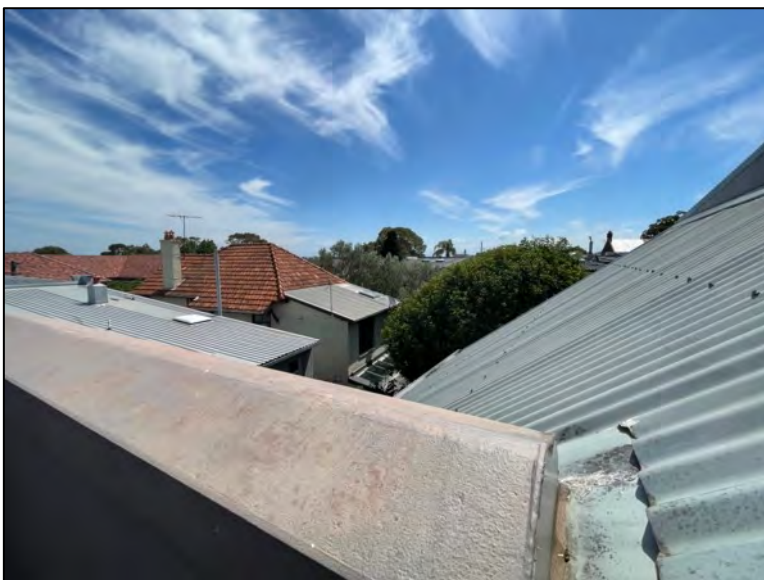
Figure 3: Rear roof No. 2 Waiwera Street looking west from rooftop.
