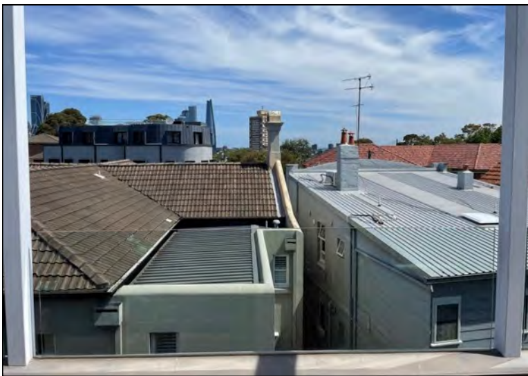
Figure 11: View from No. 2 Waiwera Street rooftop, looking south.
