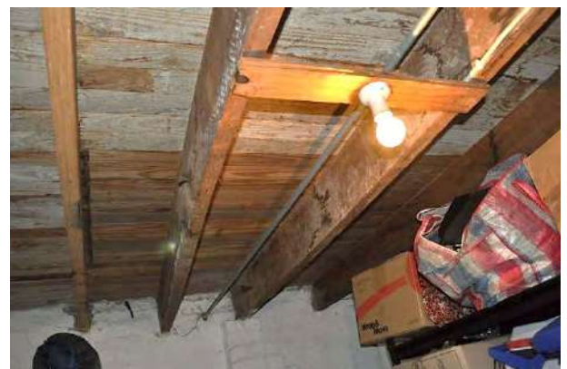
12. Mezzanine floor structure.
