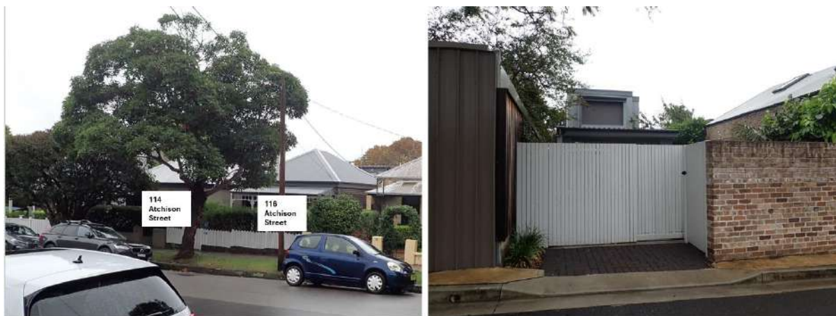
Figures 27 & 28 – Photo of site and adjoining property (left) and photo of two storey built form visible from Chandos Lane (right)
