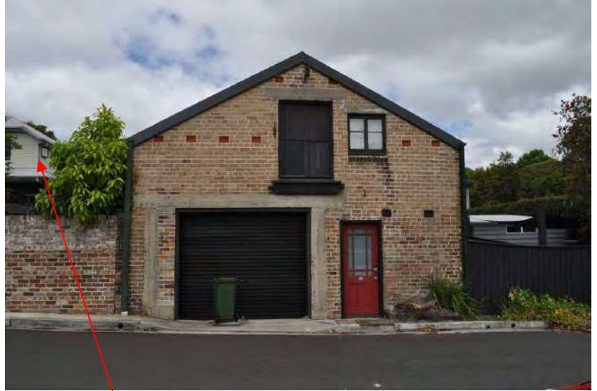
8. Rear upper level addition to adjoining house. The barn from opposite.
