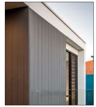
New External Walls ( FC Cladding)
