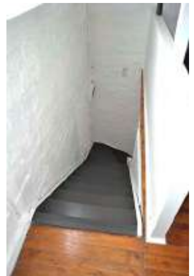
21. Stair from above.
