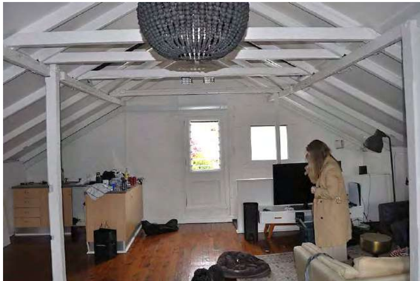
20. South wall and gantry opening.
