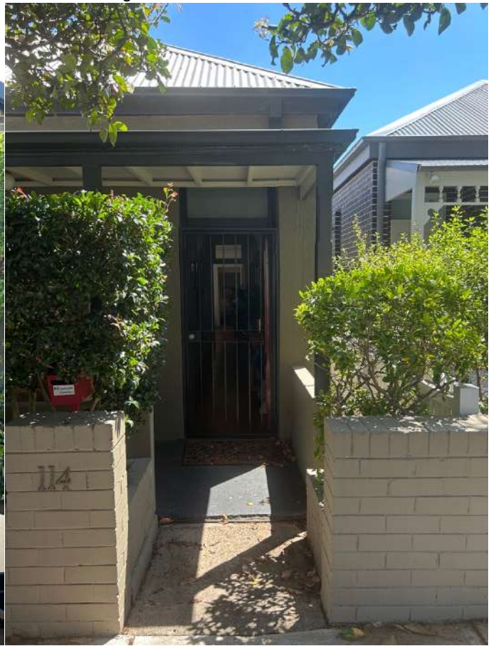
4. View of existing Entry to Dwelling off Atchison Street.
