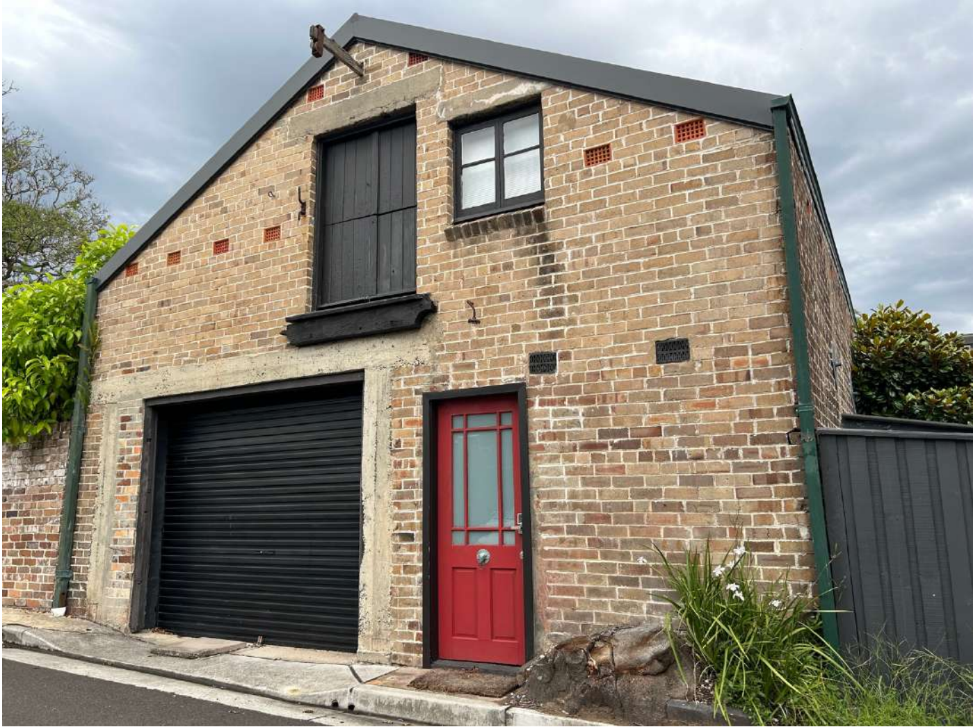
Figure 2B: Rear 'Barn' viewed from Chandos Lane
