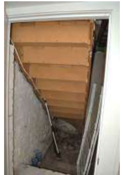
14. Underside of stair- chipboard.
