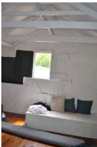
18. Roof structure and gantry.
