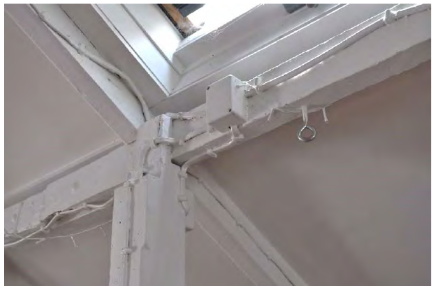
19. Roof structure posts and beams.
