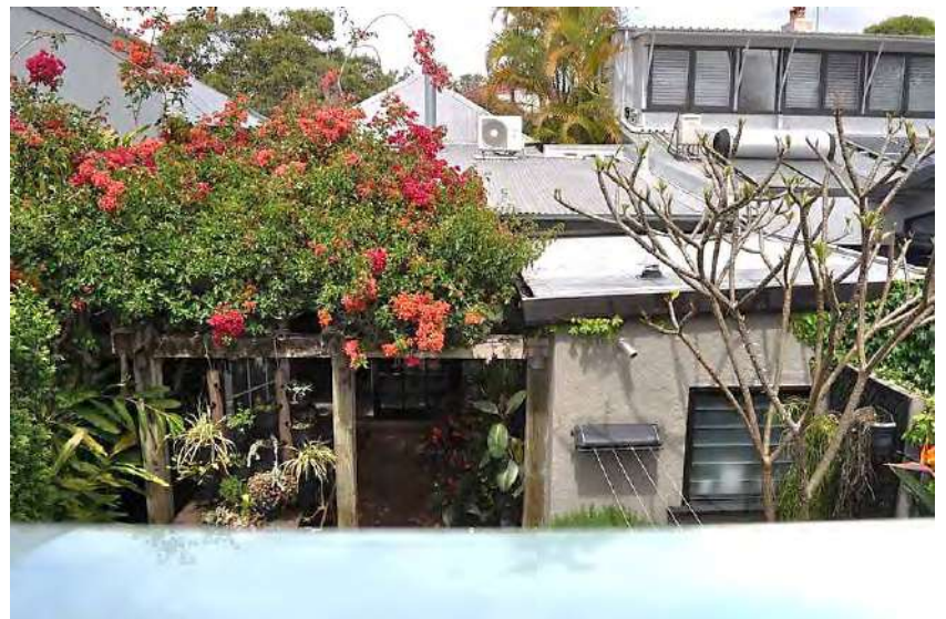
23. Rear of the house from gantry opening..
