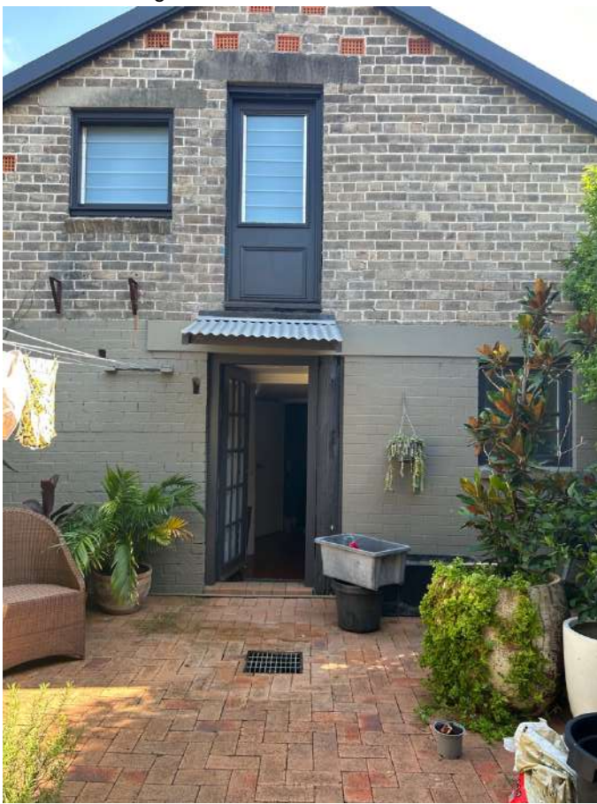
3. View of existing Barn from rear.
