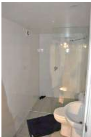
22. Bathroom to ground floor.
