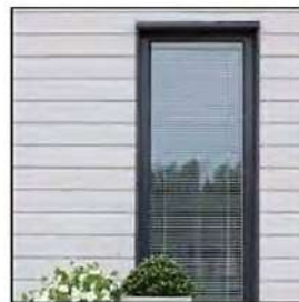
New Windows & Doors
