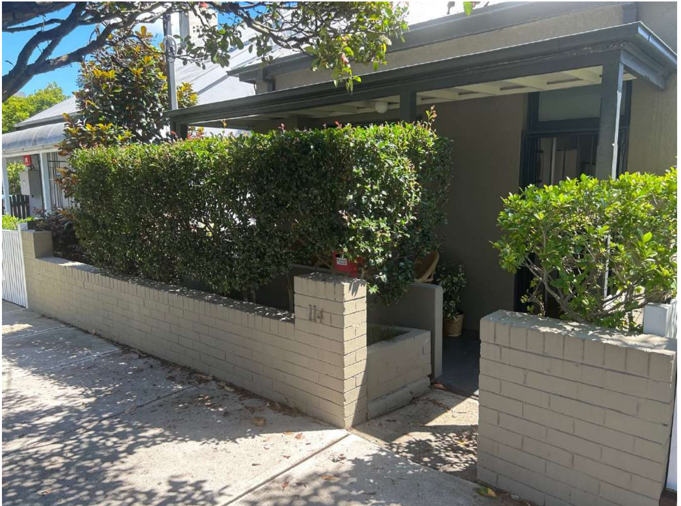
Figure 2A: The Site viewed from Atchison Street
