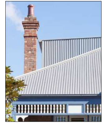
New Roof (Corrugated Steel)
