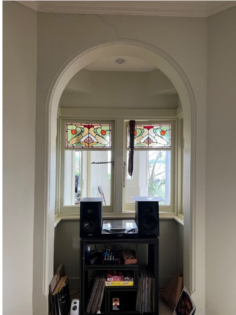
Figure 33 - Retained original alcove, including arched opening and decorative leadlight windows and timber joinery.
