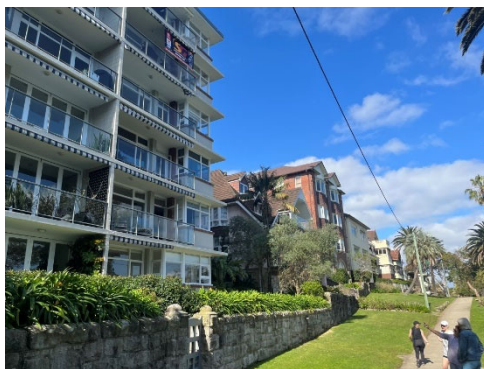
Figure 20 - View south along the foreshore reserve footpath.
