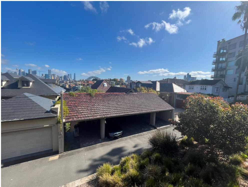
Figure 24 - View of the rear presentation of the building. The garage extends across the site, providing for three car spaces and the entry. The structure is open, with a later timber shingled clad wall below a terracotta tile roof. The roof, with later terracotta tile cladding, can be seen beyond the garage roof.
