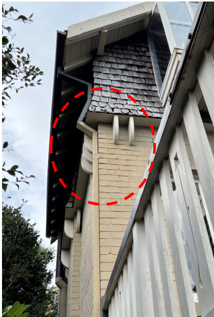
Figure 56 - Schedule of external finishes. Note the timber detailing to the balustrade as well as the timber brackets to the gable and verandahs. These details have been reconstructed based on existing building elements, see below.
