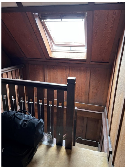
Figure 39 - Detail image of the stair and balustrade to the Attic space.
