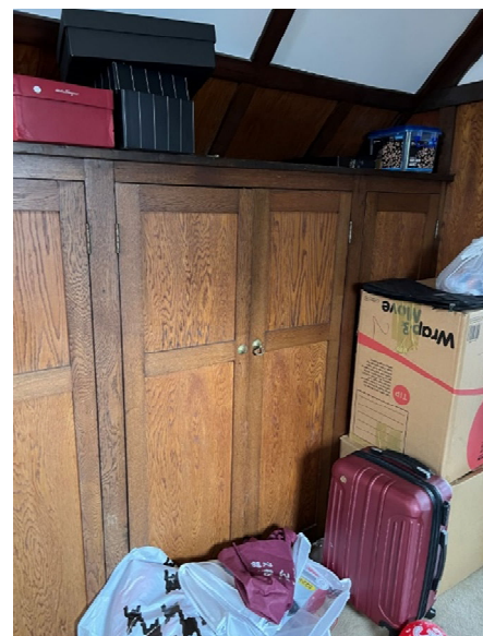
Figure 40 - Image of a built in cupboard on the stair landing.
