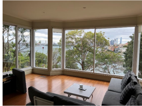
Figure 34 - Interior view of the later oversized bay window, later ceiling and floors.
