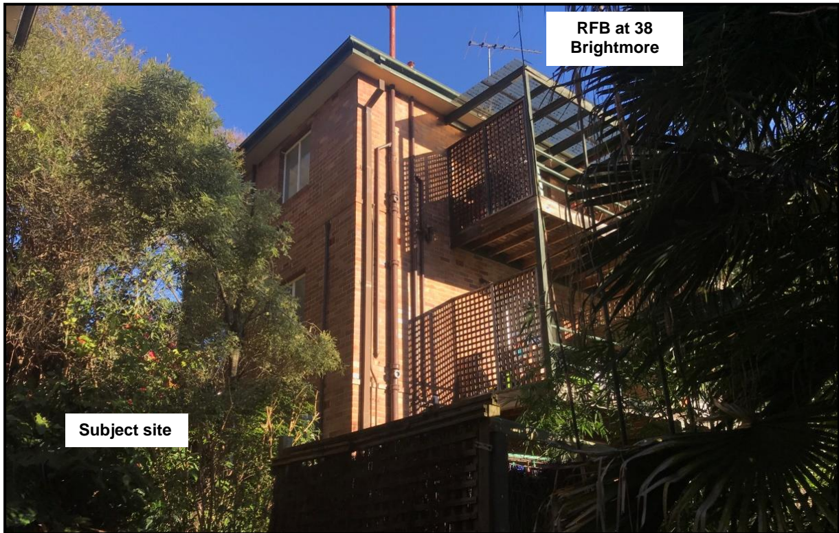
Figure 7: Rear of RFB at 38 Brightmore Street, where private open space is oriented to the north and set in from the main built form, away from the eastern boundary. Privacy screens are also located on the eastern side of the POS.
