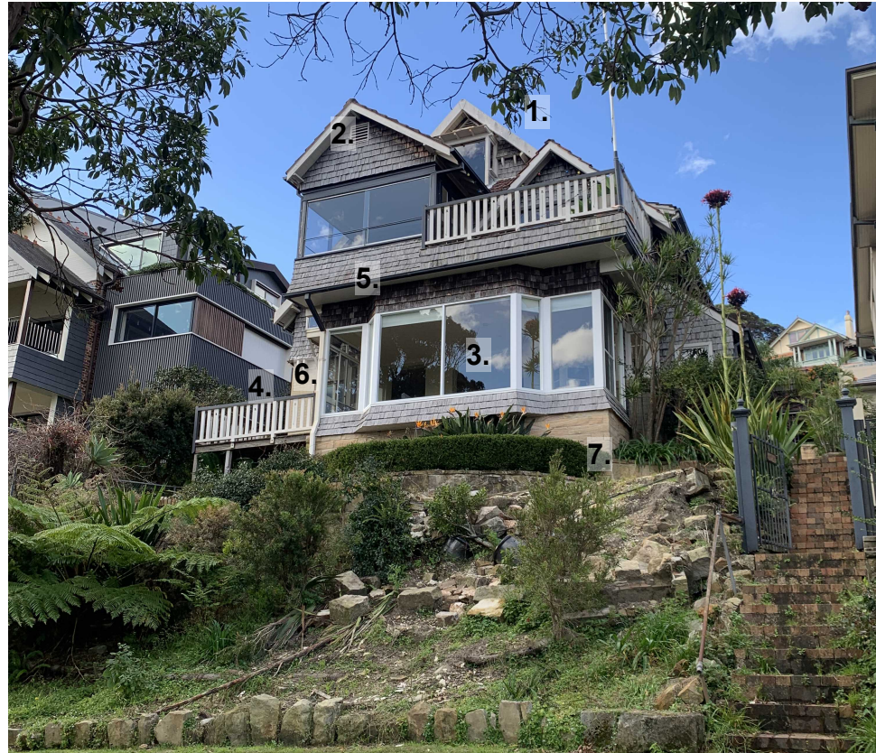
02 CURRENT PHOTO OF THE BUILDING - 2023 scale 1:NTS
