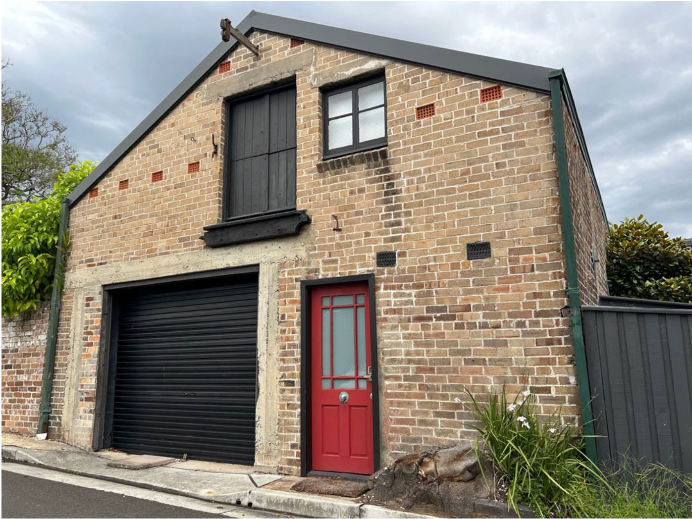
Figure 2B: Rear 'Barn' viewed from Chandos Lane
