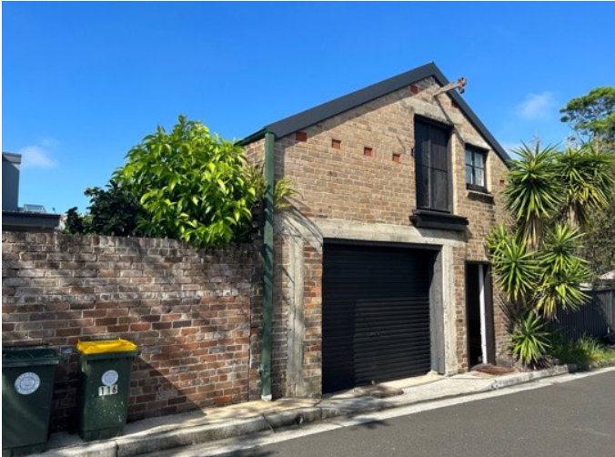
1.View of existing Barn from rear Chandos lane.
