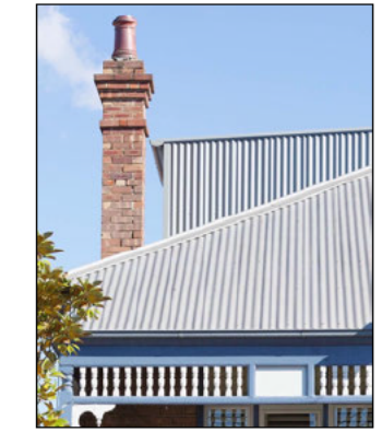
New Roof (Corrugated Steel)
