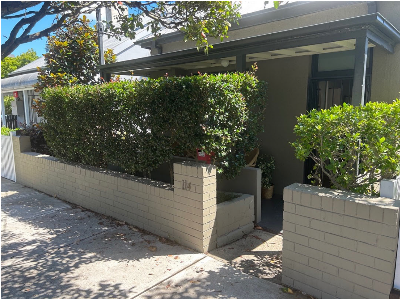
Figure 2A: The Site viewed from Atchison Street
