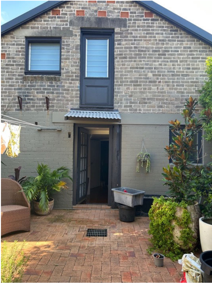
3.View of existing Barn from rear.
