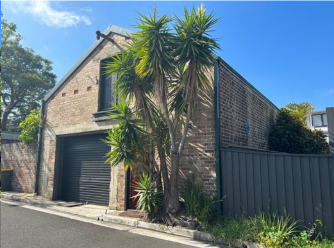
2.View of existing Barn from rear Chandos lane.
