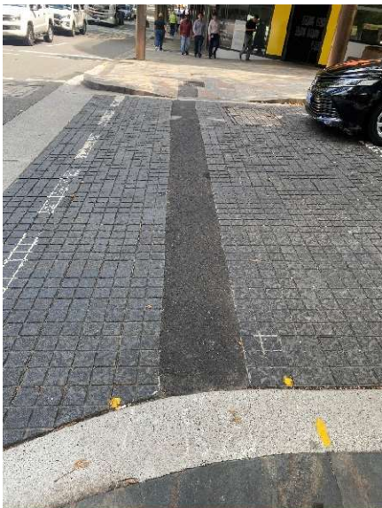
Photo 1 – restoration of trench across Mount St
