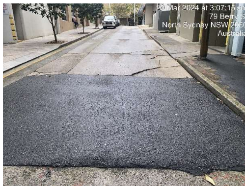
Photos – typical images of failed road sections to be reconstructed
