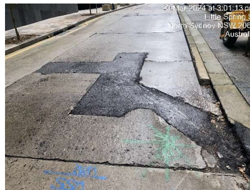
Photos – typical images of failed road sections to be reconstructed
