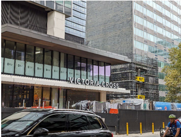
Picture 3 Victoria Cross Station from Miller Street
