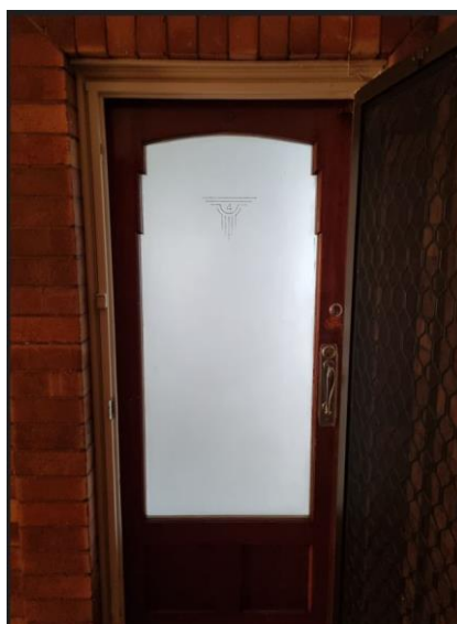
The original glazed apartment entry doors will be replaced.
